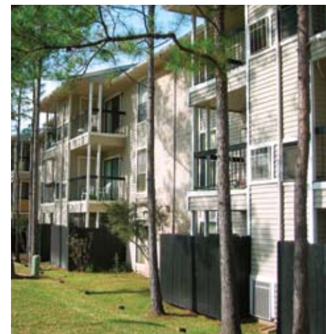
Copperwood Apartments Houston, TX
