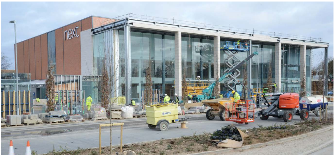
High Wycombe – Under construction February 2015
