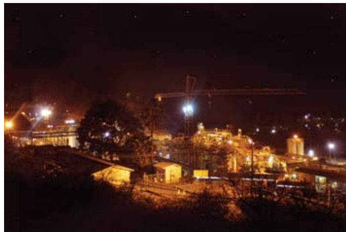
BIOX® plant at night - Fairview
