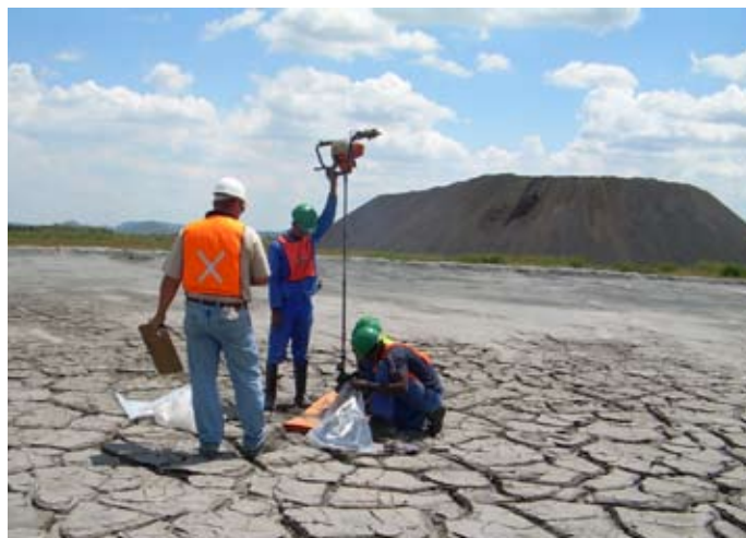
Auger drilling taking place on top of tailings dam
