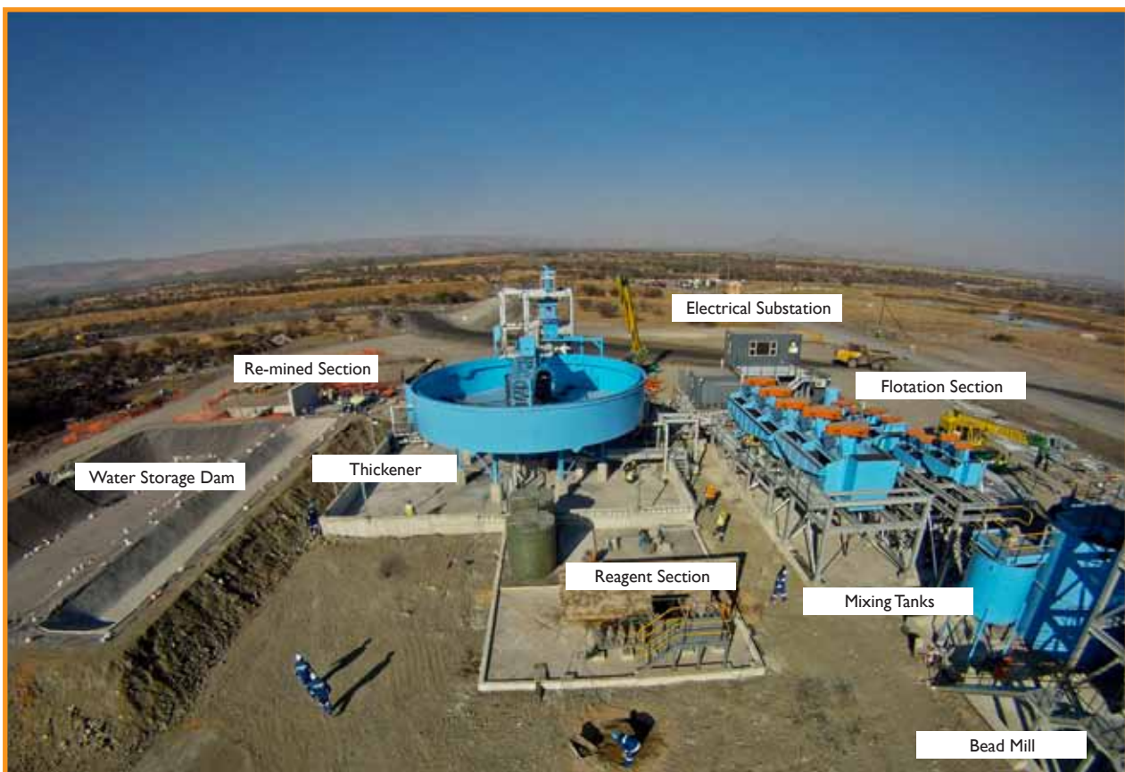
Plant Construction as at August 2011.
