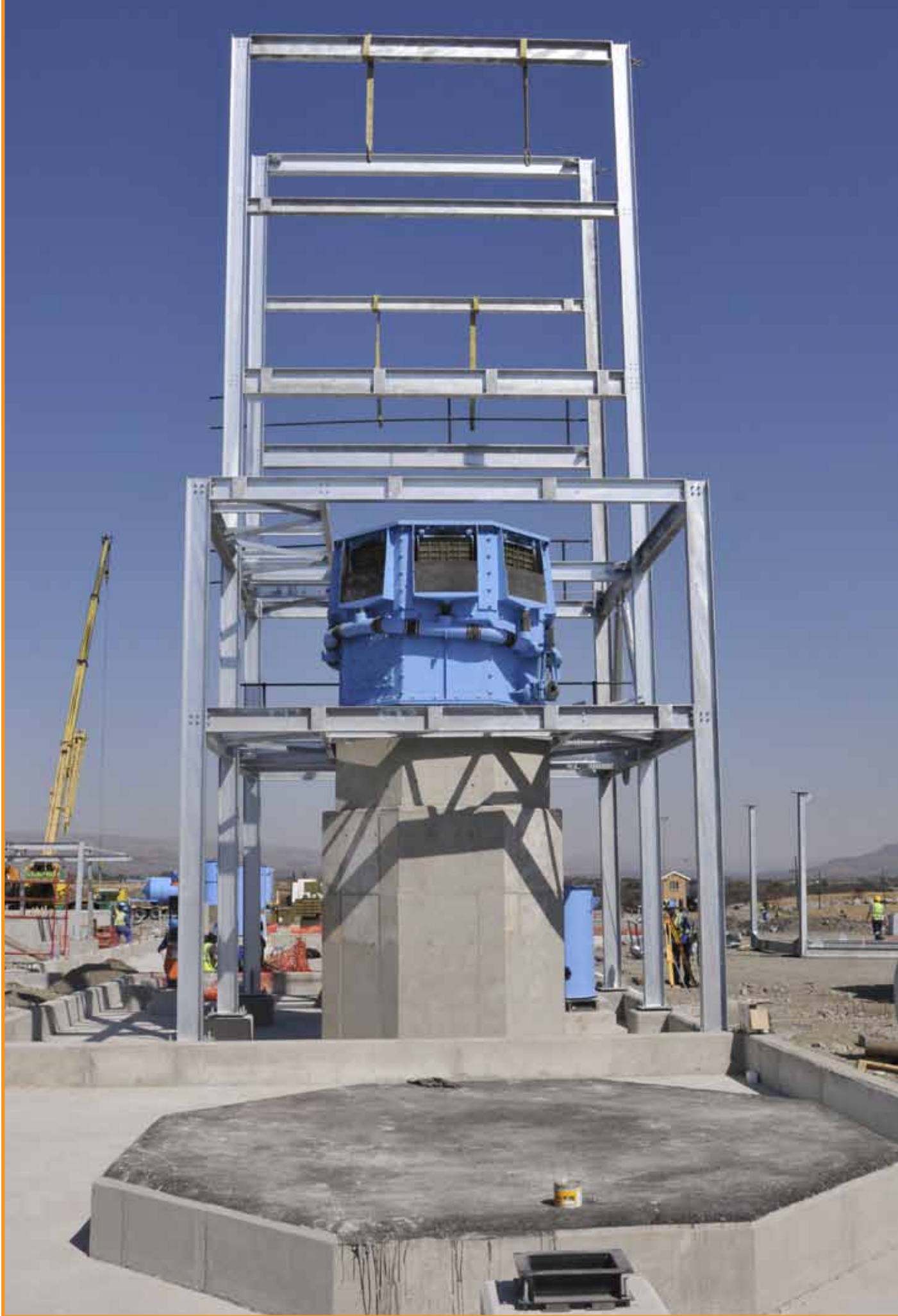
Phoenix Plant Construction.
