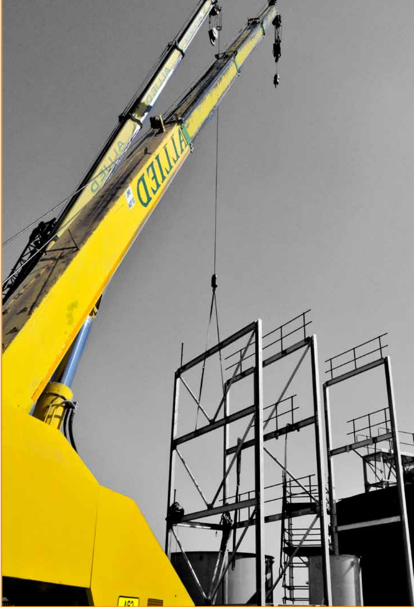
Plant Construction, Phoenix Platinum
