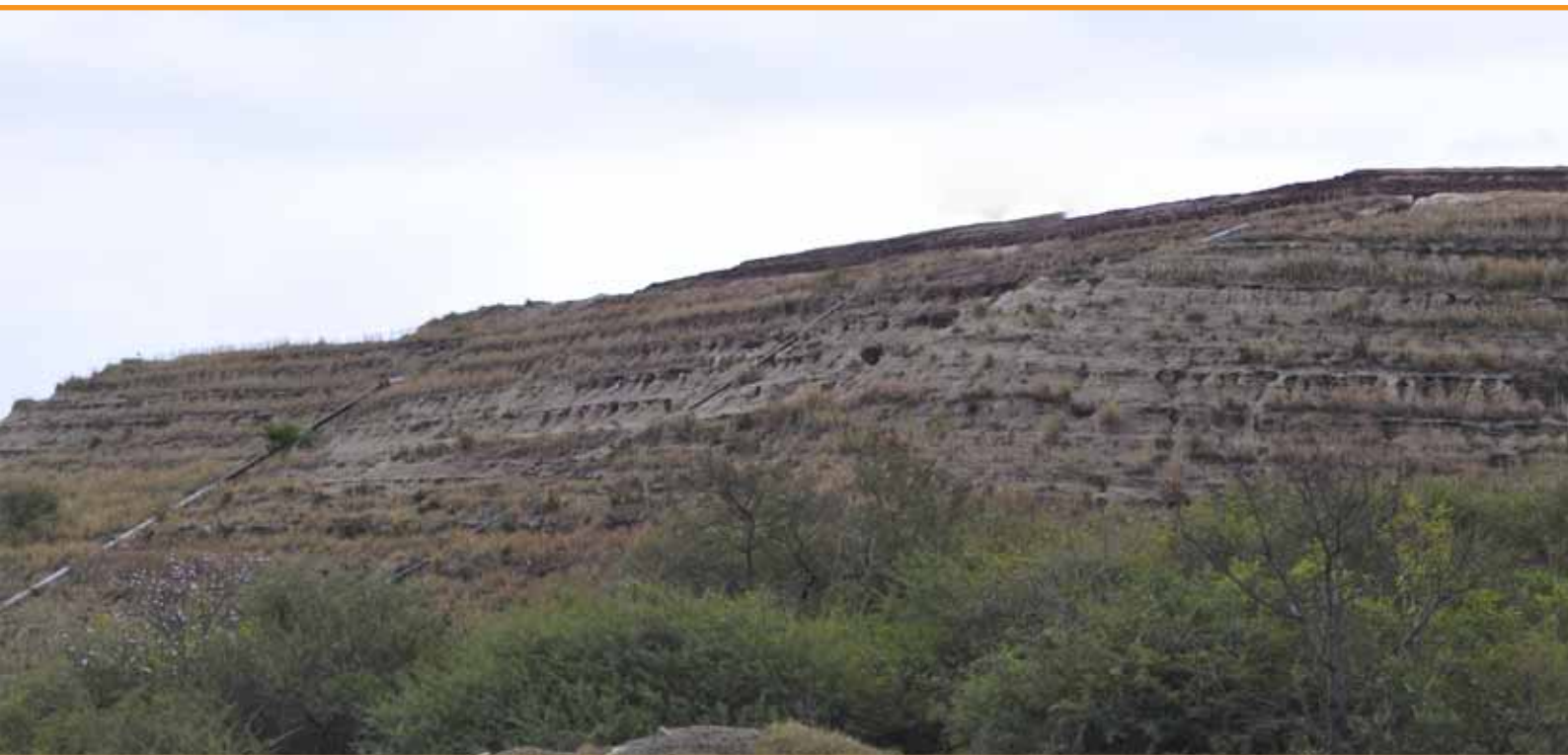
Harper Tailings Dam, Barberton Mines.
