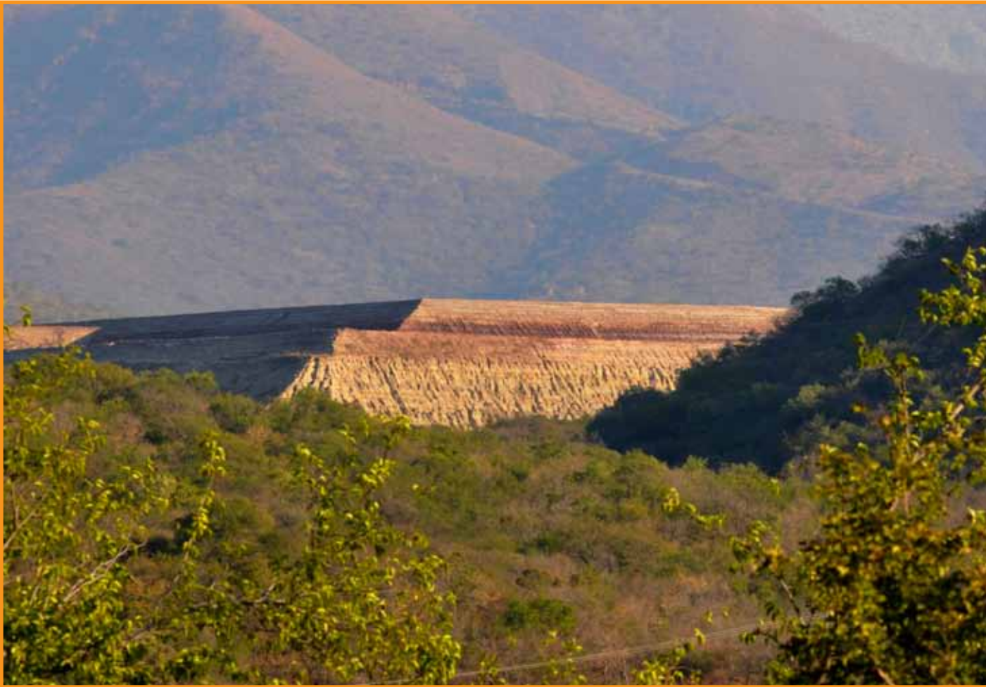
Harper Tailings Dam, Barberton
