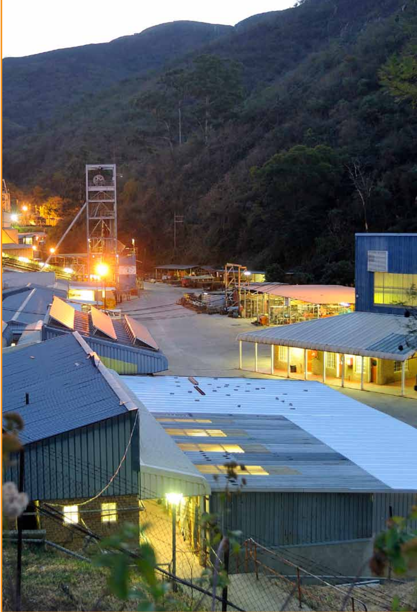
Headgear, Sheba Mine
