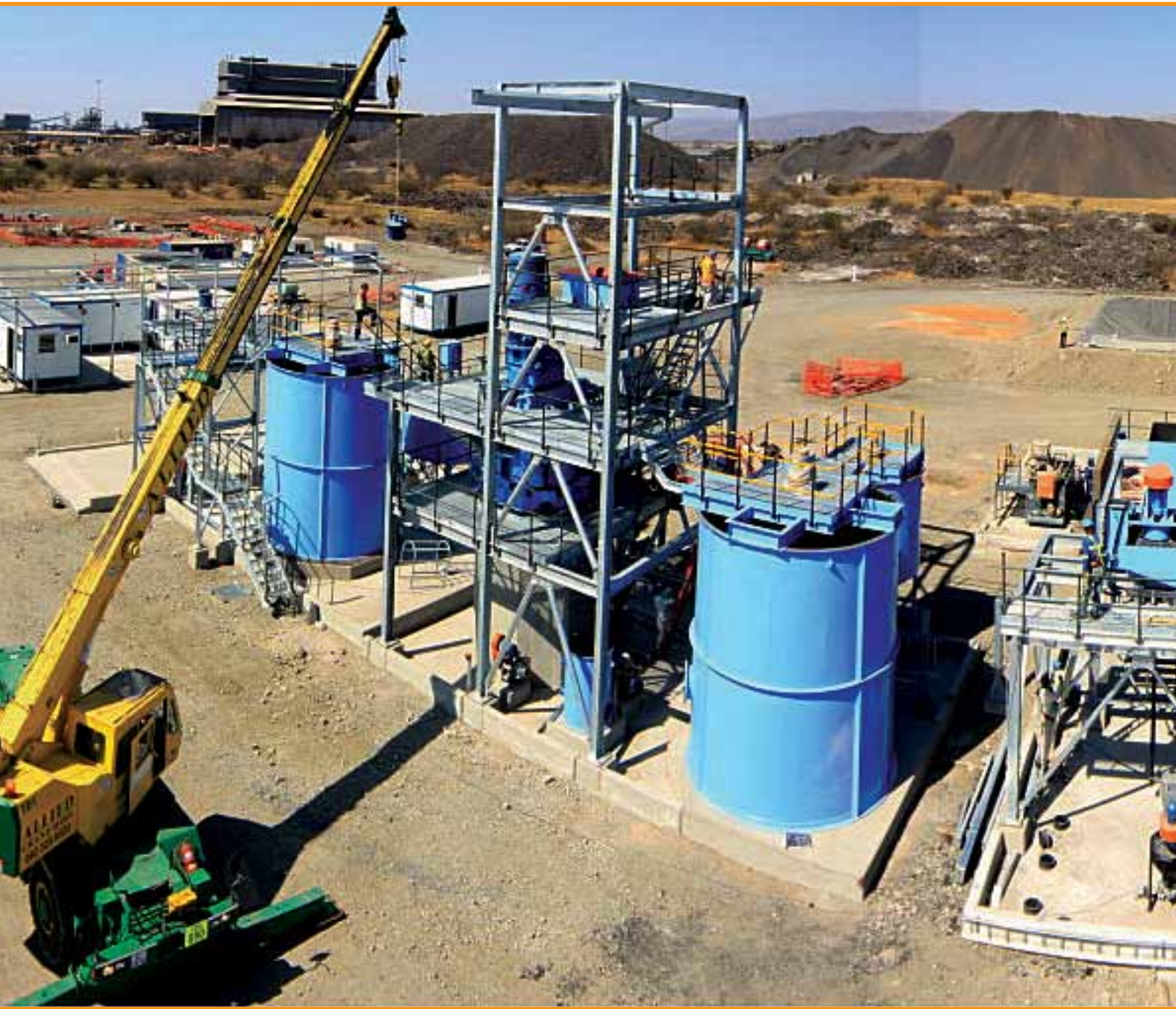
Phoenix Platinum, plant construction progress as at August 2011.
