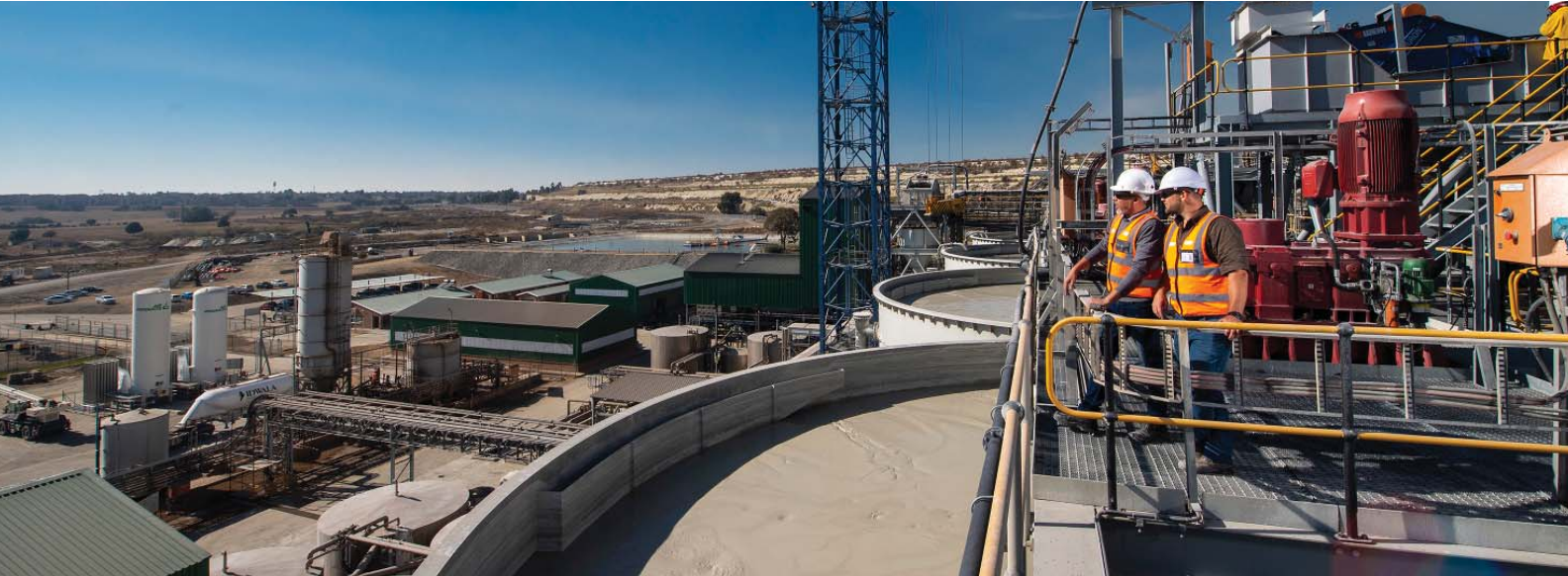
▼ Elikhulu plant – inspecting CIL tanks
