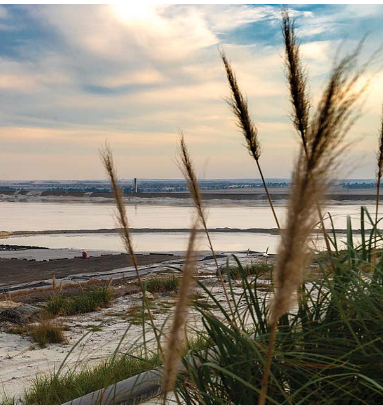
< Elikhulu – TSF – deposition of tailings
