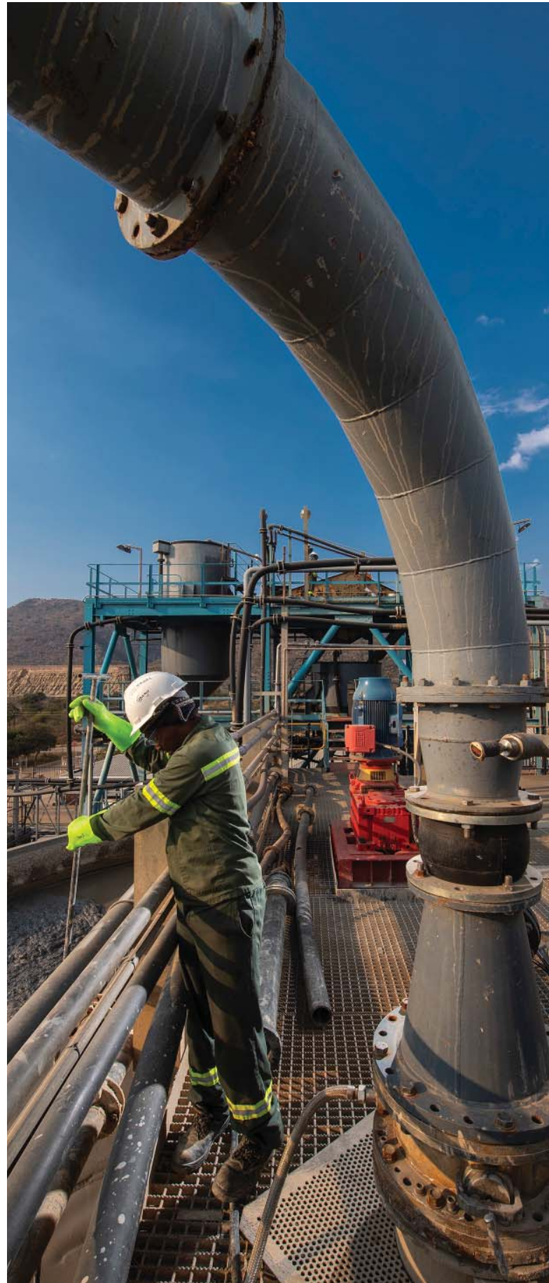
▼ Barberton Mines – BTRP plant
