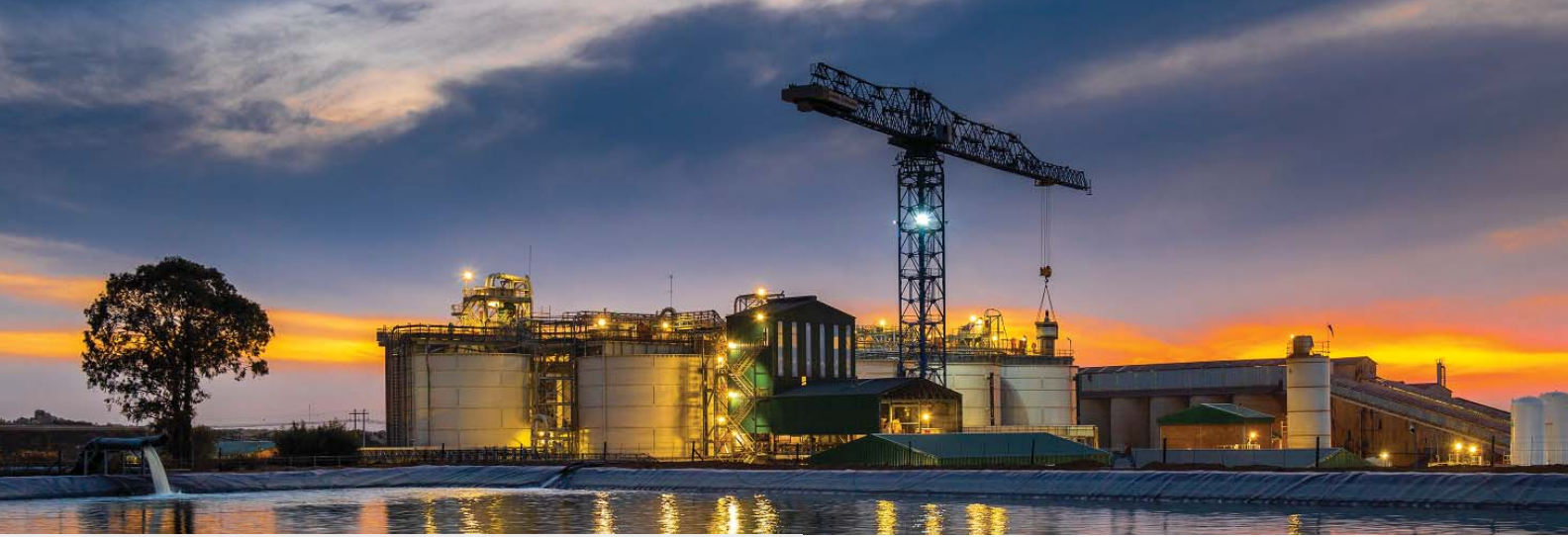
▼ Elikhulu Plant – process water dam in foreground
