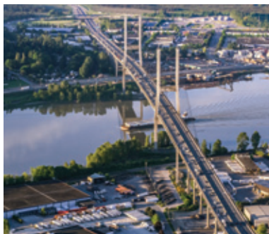
High-profile Road Zipper contracts awarded in 2018 include the Alex Fraser Bridge in Vancouver, British Columbia, Canada and The Richmond-San Rafael Bridge in San Francisco, California.
