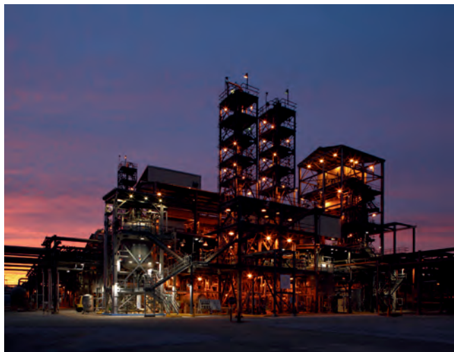
FMC acquired 14 production sites worldwide as part of the DuPont transaction, including this state-of-the-art active ingredient manufacturing facility located near Mobile, Alabama.
