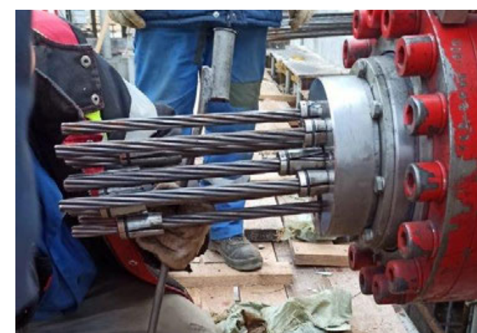
Installation of a large-span slab with prestressed reinforcement
