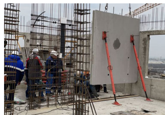
Assembly of prefabricated reinforced concrete walls as part of cast-in-place construction
