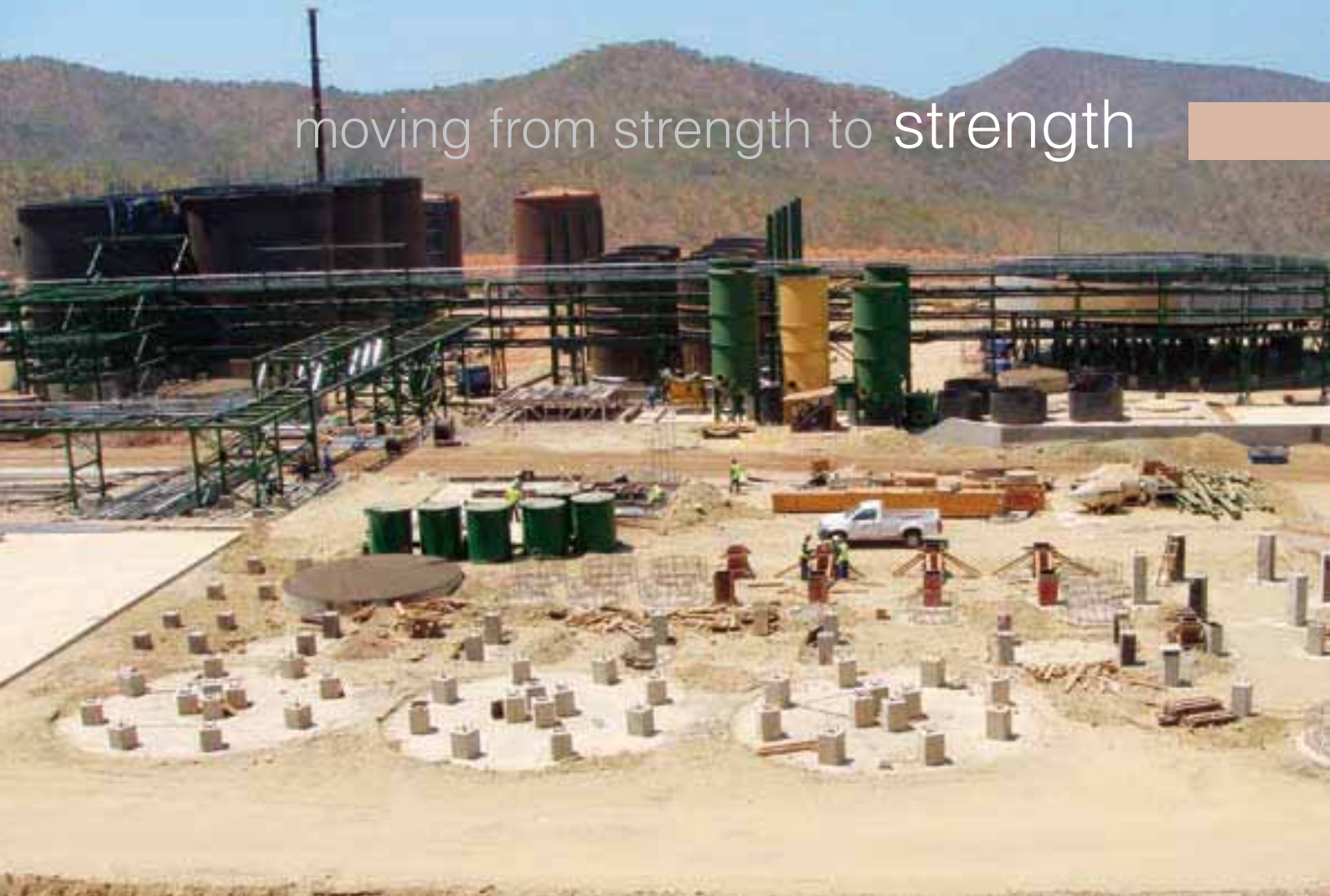
Pictures left to right: (1) and (2) Kayelekera
