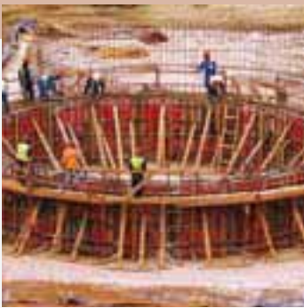
In Construction Kayelekera
