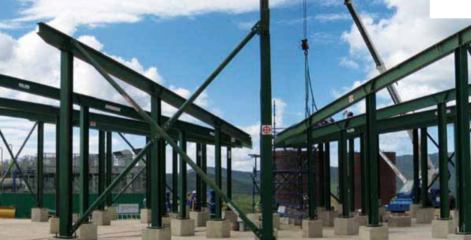
Pictures left to right: (1) and (2) Kayelekera
