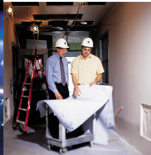
Scott Wheelwright, Vice President of Manufacturing, and Jason Brenner, Facilities Manager, discuss the construction plans for the commercial manufacturing facility.
