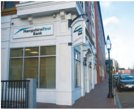
The Portsmouth Office of Hampshire First Bank is located a few blocks from the Atlantic shoreline.
