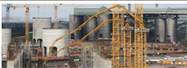
Typically are used for high-rise projects and can be mounted upon a self-rising mount or base
