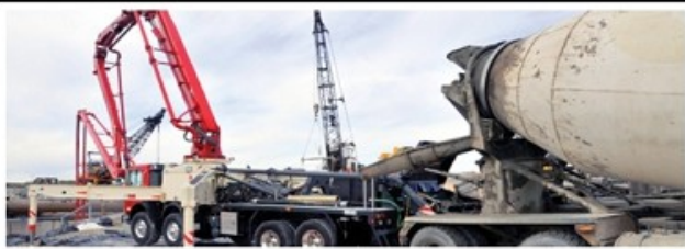
Mobile, truck-mounted boom pumps with vertical reach of over 200 feet
