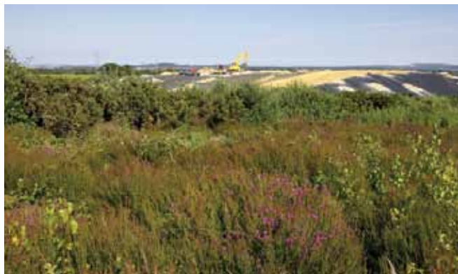
Trigon landfill restoration, Dorset.
