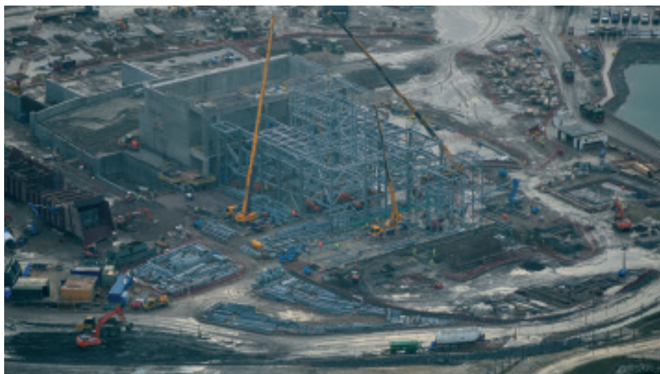
Ardley EfW, Oxfordshire, under construction
