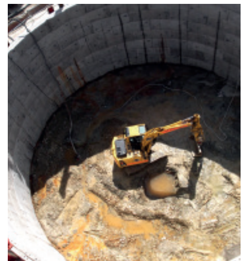
Construction of storm storage tank at Lostwithiel, Cornwall
