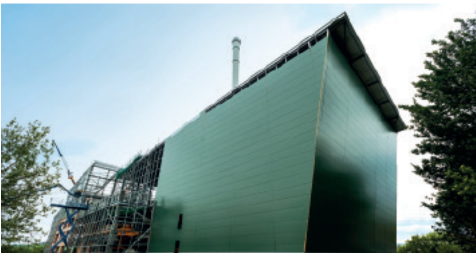
EfW facility, Exeter, under construction
