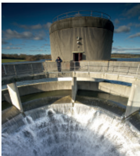
Spillway at Roadford Reservoir, Devon
