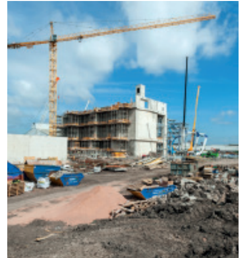
Trident Park EfW, Cardiff, under construction
