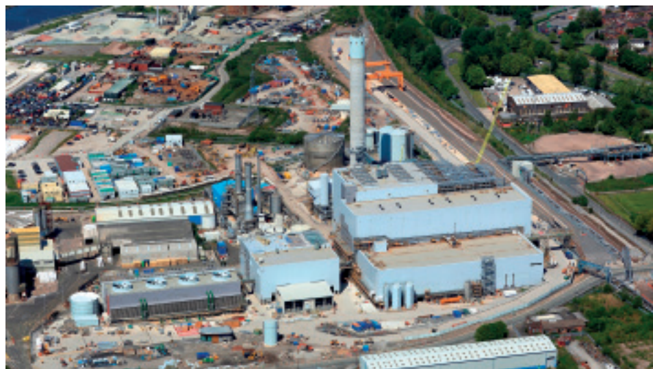
EfW/Combined Heat and Power (CHP) facility, Runcorn, under construction
