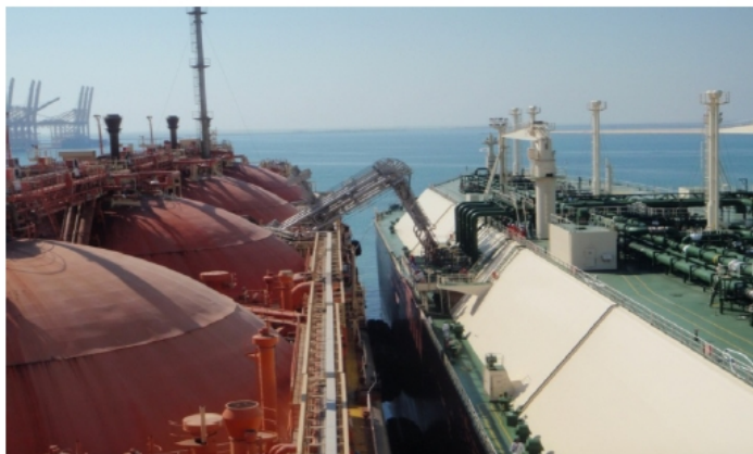
Golar FSRU, Golar Freeze, receiving cargo from Qatargas LNG Carrier in Dubai
