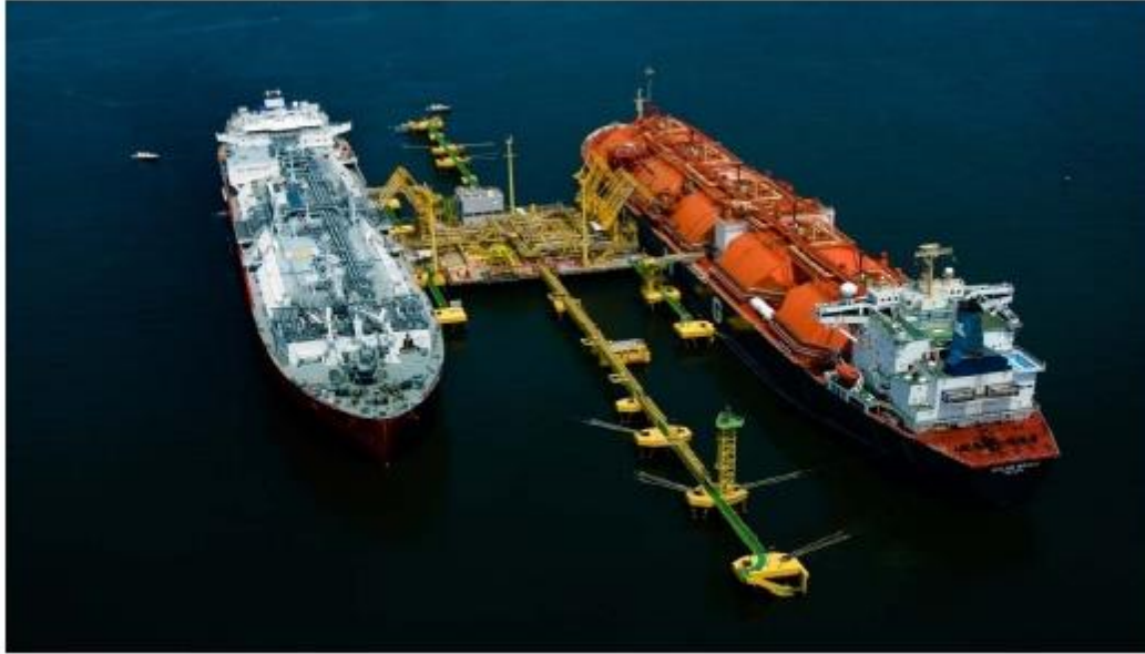
Golar Spirit FSRU receiving cargo from LNG Carrier in Guanabara Bay, Rio de Janeiro
