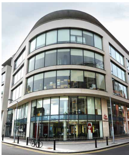
The Chancery 3 - 10 Chancery Lane, Dublin 8
