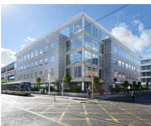
New Century House, Mayor Street, IFSC, Dublin 1
