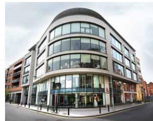
The Chancery, 3 – 10 Chancery Lane, Dublin 8
