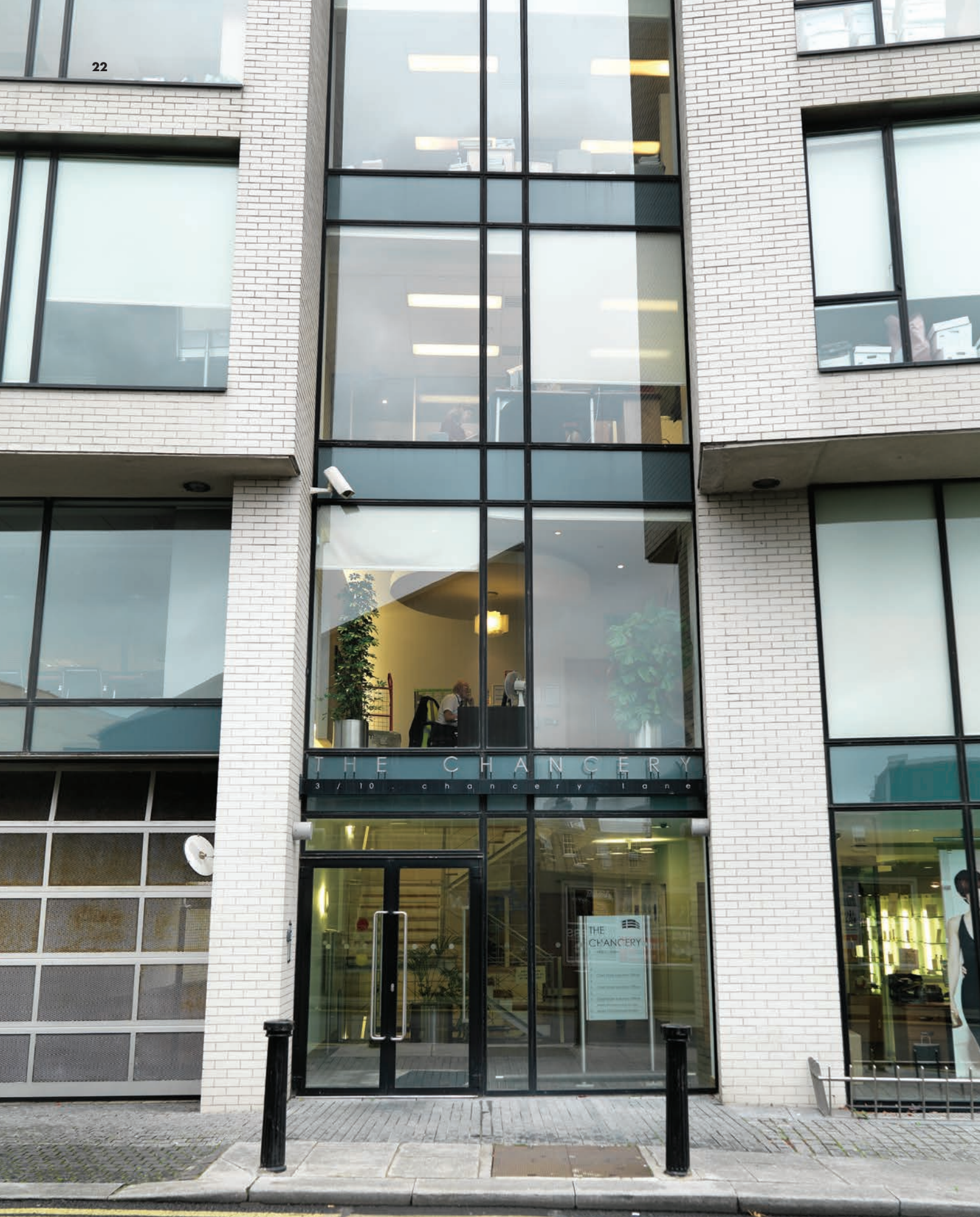
Chancery Building Chancery Lane Dublin 8
