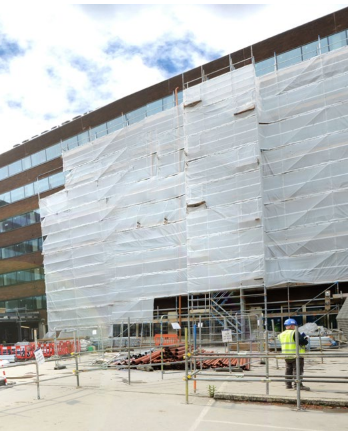
Photograph of the building works at Cumberland House, Dublin 2
