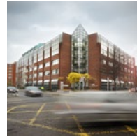
15. 1 Earlsfort Terrace Dublin 2
