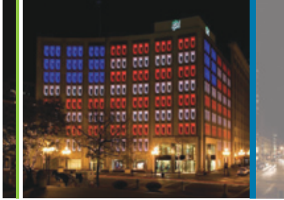
Indianapolis Power & Light, Indiana
