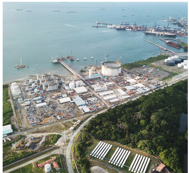
380 MW Colón (CCGT/LNG regasification and storage facility, Panama)
