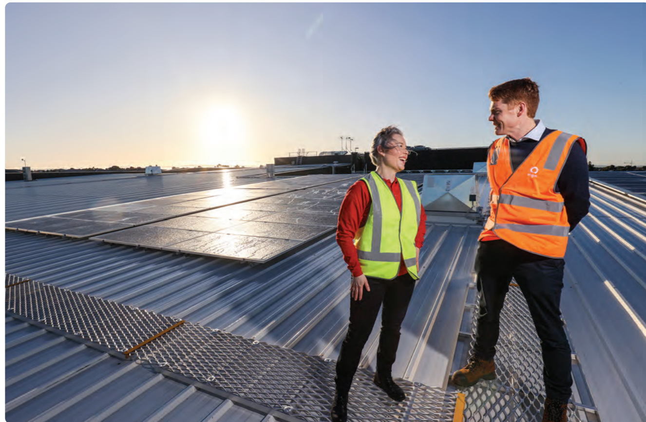
Pictured: Head of Energy Jane Mansfield and Origin Zero Executive General Manager James Magill inspect the rooftop solar panels at Coles Craigieburn Village, following a landmark agreement to co-invest energy and battery assets.
