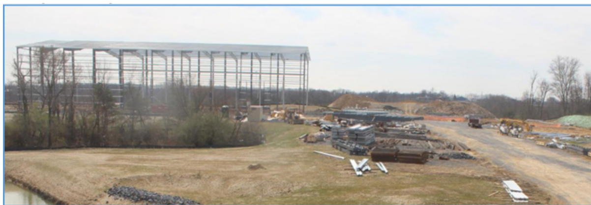
Entsorga West Virginia Plant Under Construction – March 2017
