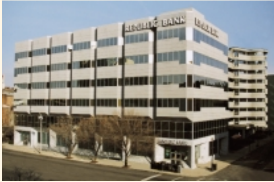
REPUBLIC BANK CORPORATE CENTER 601 W. Market Street, Louisville
