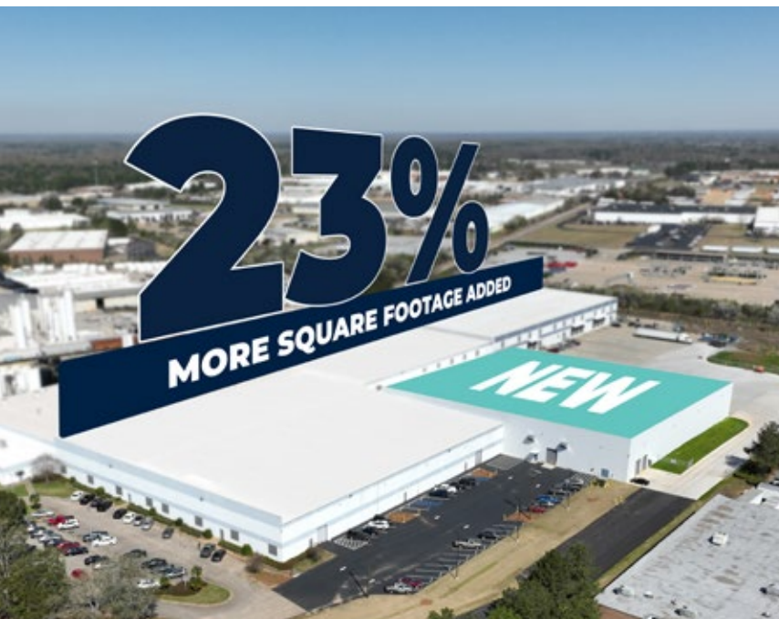
Kinpak, Inc. - Manufacturing plant in Montgomery, Alabama.
