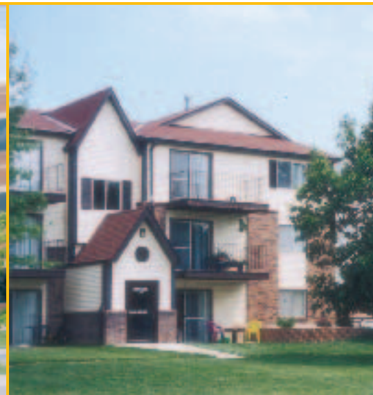
Thomasbrook Apartments • Lincoln, Nebraska
