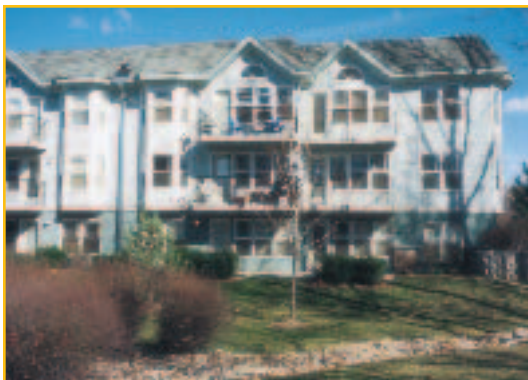
Clearwater Apartments • Boise, Idaho
