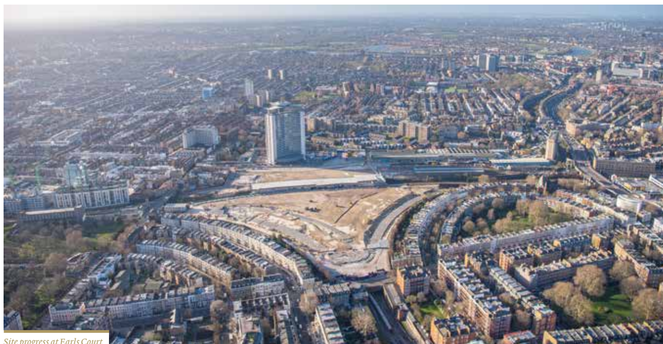
Site progress at Earls Court
