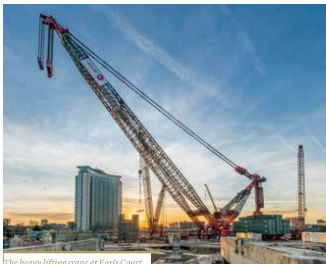
The heavy lifting crane at Earls Court
