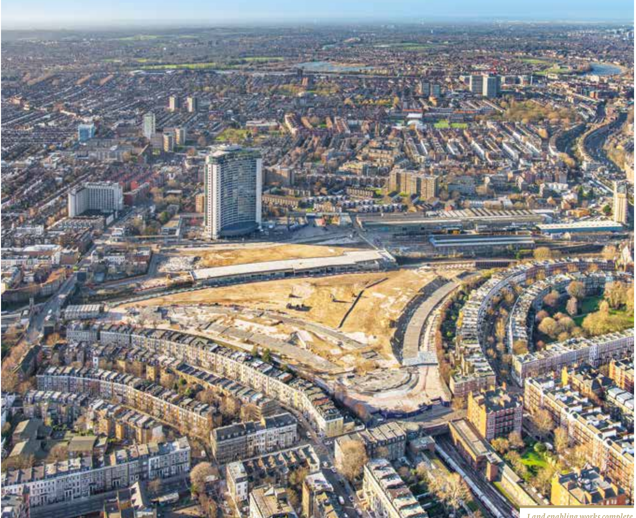
Land enabling works complete
