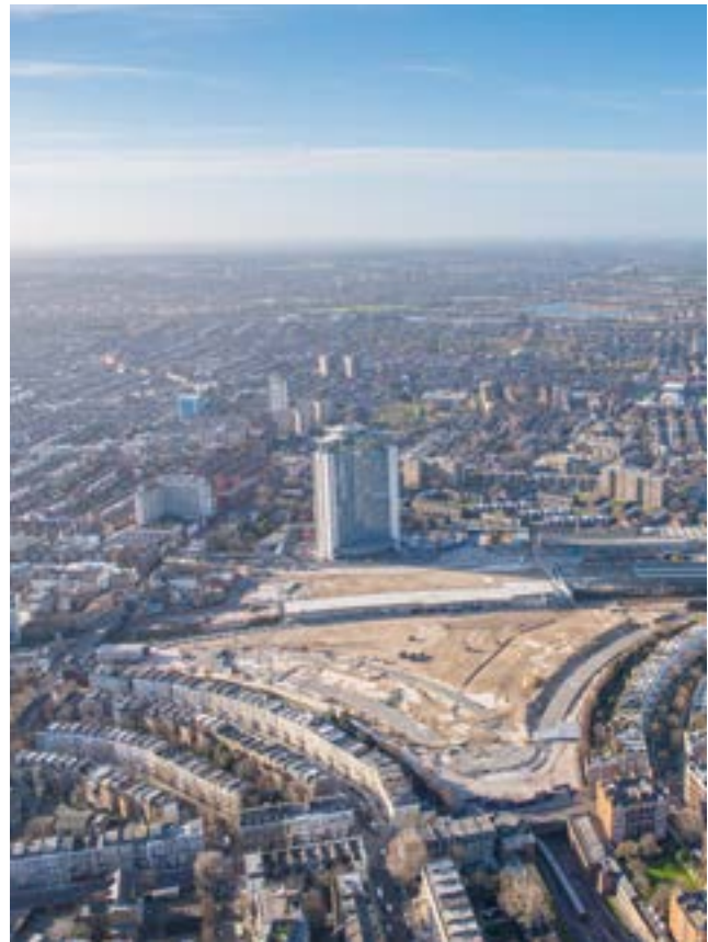
Site progress at Earls Court
