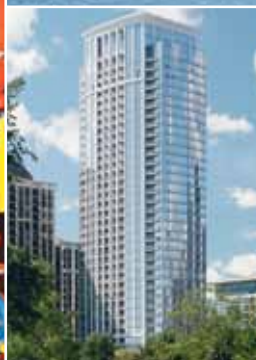
Energy efficient heating, ventilation, and air conditioning
