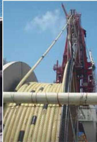
Perma-Pipe Gulf of Mexico installation
