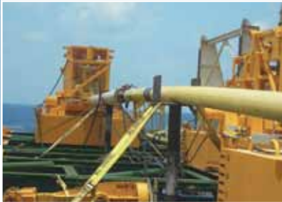
Perma-Pipe submerged piping installation
