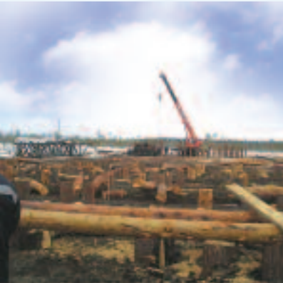
Pile Driving for Lineynoye 7 Rig Platform
