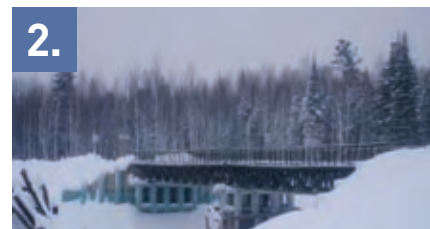
1. Kiev-Egan bridge under construction. 2. Completed bridge.
