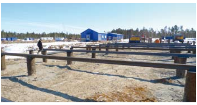
Field facilities under construction at Lineynoye.
