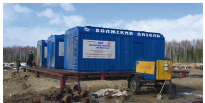
Modules of the Gas Powered Piston Plant which will utilise associated gas to provide power for field operations thereby eliminating the need to flare gas.
