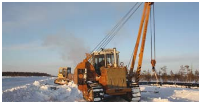
Laying out the pipe for construction of the Lineynoye-Kiev Eganskoye pipeline.
