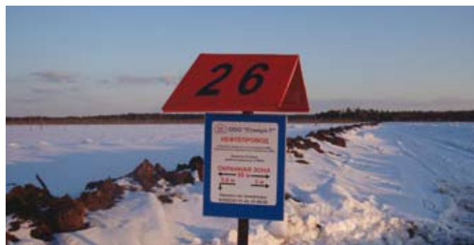
Distance marker along the completed pipeline route.
