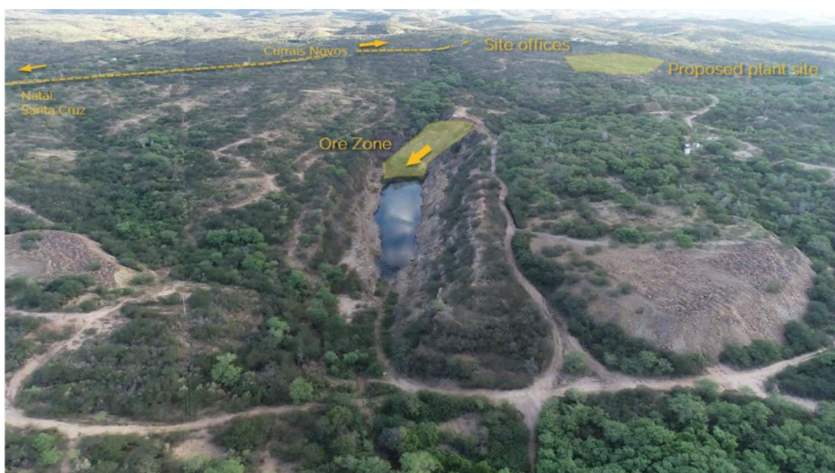
Figure 3. View to the south west over Borborema pit showing exposed ore zone and infrastructure – existing and designed.
