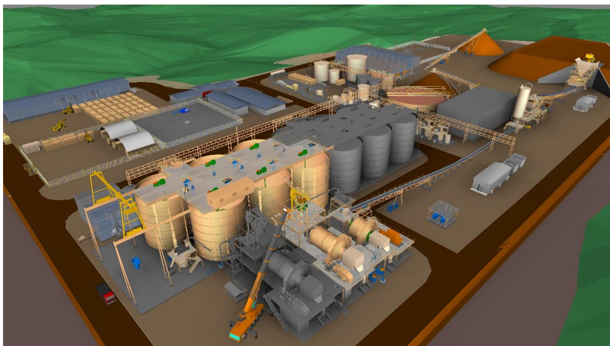
Figure 4. Borborema 2Mtpa Stage 1 plant and equipment and revised layout recommended by Option Study, showing additional plant for a possible future expansion (illustrated in grey).
