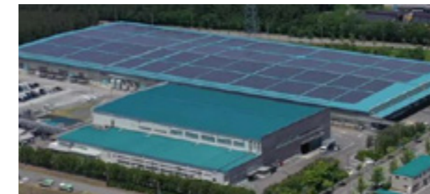
Photovoltaic (solar) power generation facilities at Sakata Plant
