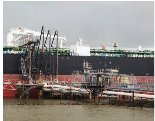
Supply ship at Caltex Fuel Terminal, Lytton
