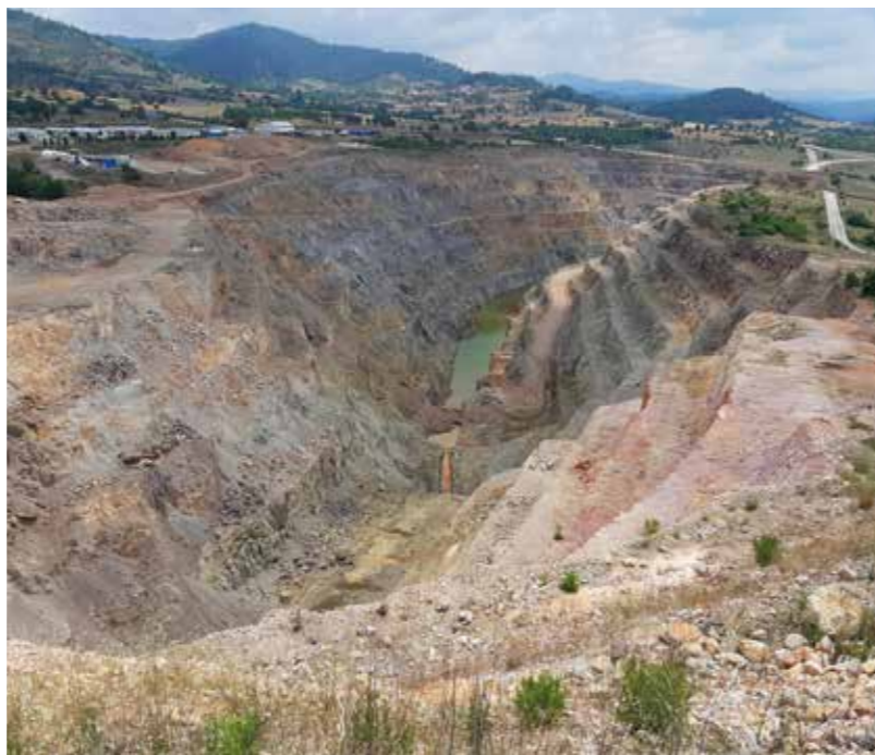
Arzu South open pit, with the Kiziltepe Mine administrative buildings shown to the left.
