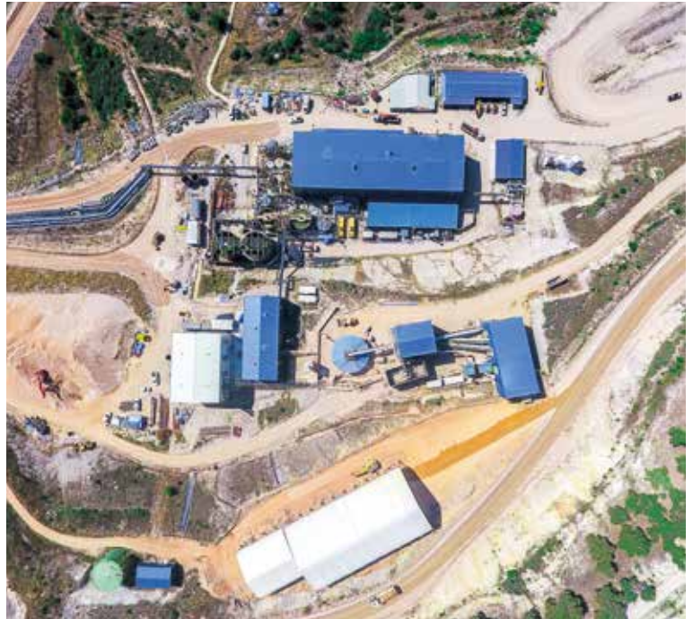
Kiziltepe Mine Processing Plant, following plant expansion in 2021.
