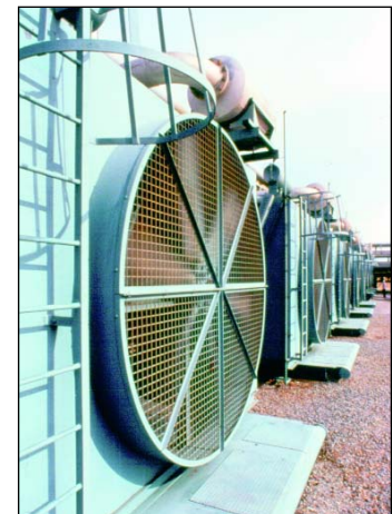
Harsco's air-cooled heat exchangers provide critical pipeline and compressor cooling for natural gas exploration and distribution locations.
