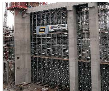
Lightweight yet structurally strong, the GASS aluminum shoring system provides heavy-duty support during construction of a new energy facility.
