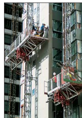
Harsco's acquisition of additional Mast Climbing Work Platforms provides customers a time-saving alternative to traditional scaffolding for certain project requirements.
