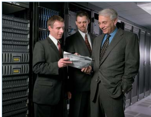
To the right, President, CFO and Treasurer Sal Fazzolari receives an update on Harsco's new High Availability Data Center from Scott Gerson, VP and Chief Information Officer (center) and Terry Stahler, Director of Global IT Infrastructure (left).
