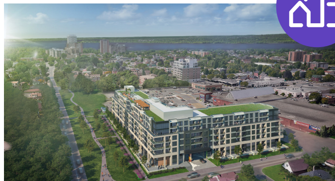
Element Ottawa, ON A unique rental community in the vibrant Westboro Village, one of Ottawa's most desirable neighbourhoods
