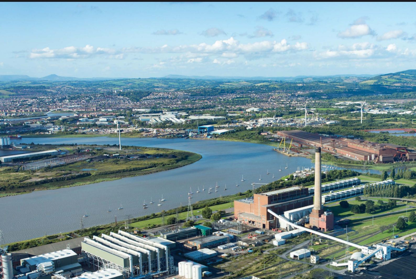
Uskmouth Power Station
