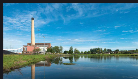
Uskmouth power station
