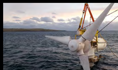
Andritz Hydro Hammerfest 1.5MW tidal turbine prepared for installation
