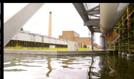
Uskmouth Power Station, view from inside of a cooling tower westward
