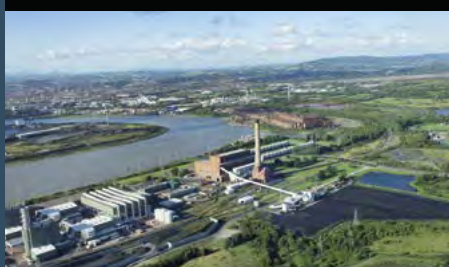
Uskmouth power station
