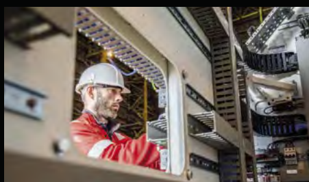
AR500 System Testing - Shop 1 Nigg Energy Park
