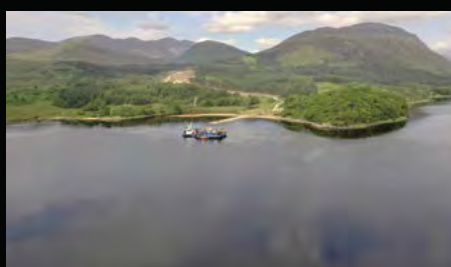
Cable laying - Loch Etive
