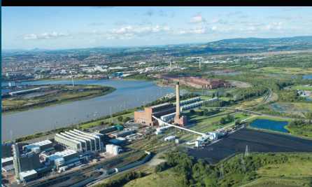
Uskmouth power station
