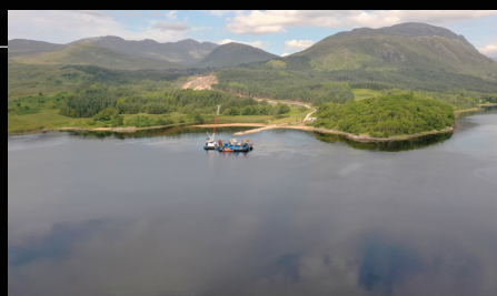
Cable laying - Loch Etive
