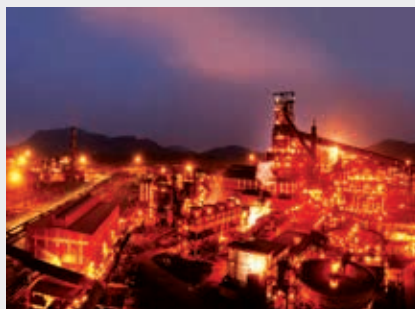
Capacity Expansion at State-of-the-art Kalinganagar Steel Plant
