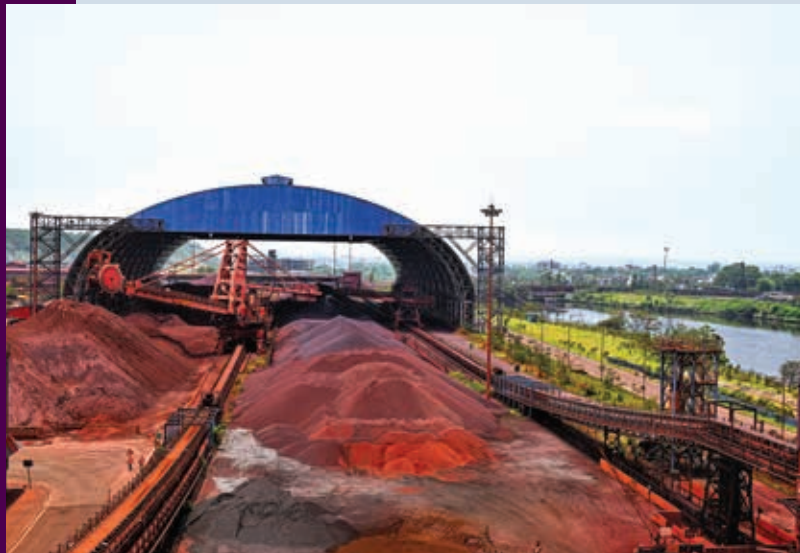
Pellet Plant, Jamshedpur Works: Achieving resource efficiency
