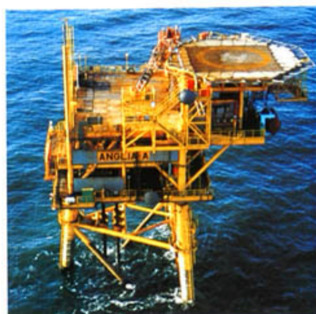
Anglia production facility, North Sea, United Kingdom.
