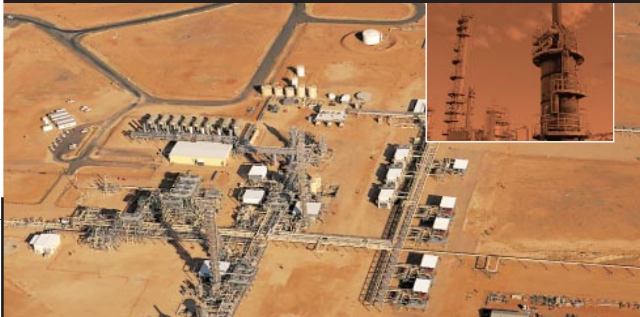
Ballera Gas Plant
