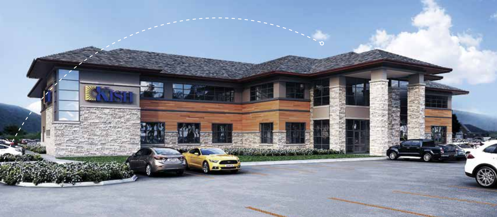
A 3-D rendering of the Kish Innovation Center, now under construction on Kish's Reedsville campus. The new 38,000-square-foot technology and operations hub will enhance employees' capacity to serve customers.
